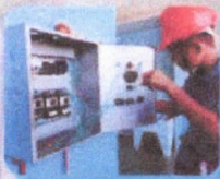
ELECTRICAL INSTALLATION & MAINTENANCE NC II & NCIII
