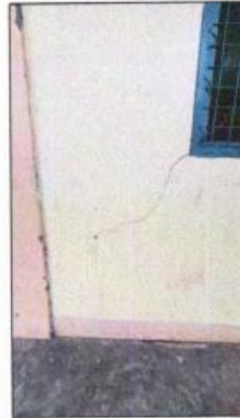
(SW-2) - REPLACEMENT DAMAGED MASONRY WALLS, 100mm THK. CHB W/ PLAIN CEMENT PLASTER, PAINTED FINISH
