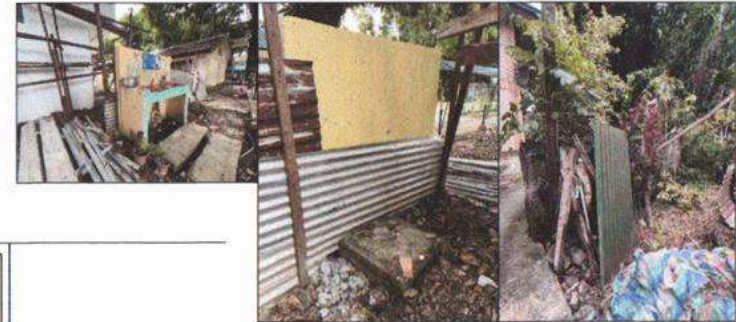
Demolition of Existing/Obstructing Structures:
