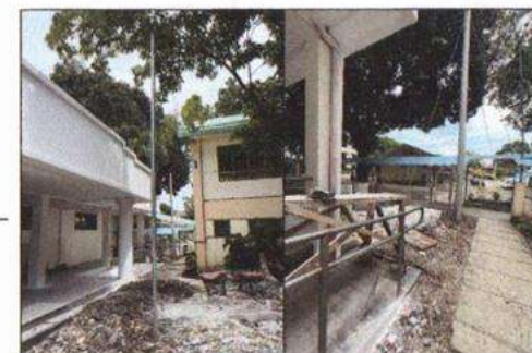
Relocation of Electrical Post and Guy Wire Pole Support:
